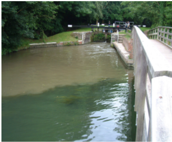
☞ Sediment problems at confluence of the Kennet and Avon Canal and the River Kennet
