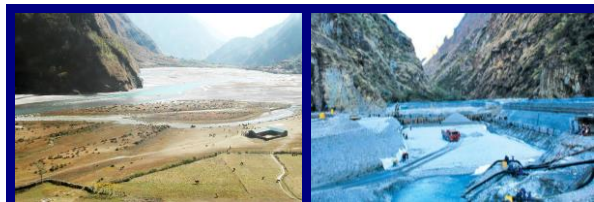
Left image: Sediment filled basin behind historical landslide.
