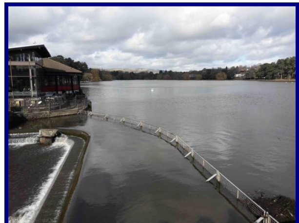
Figure 3 Roath Park ornamental lake, looking upstream from the spillway
