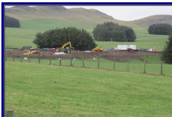
Figure 5. Preliminary construction work for the windfarm development
