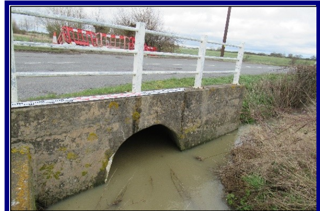
Existing culvert under the East Hanney-Steventon road.
