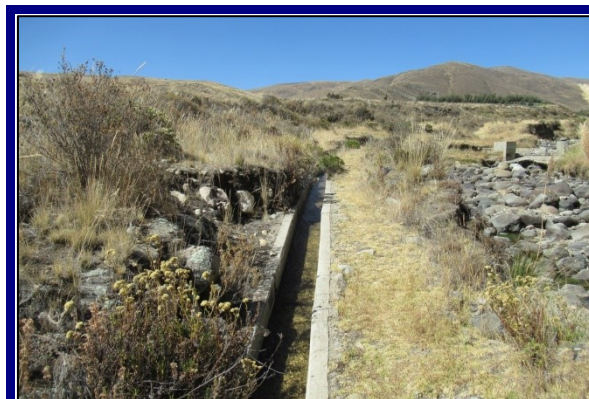
Figure 3 Irrigation canal in the Cordillera Negra
