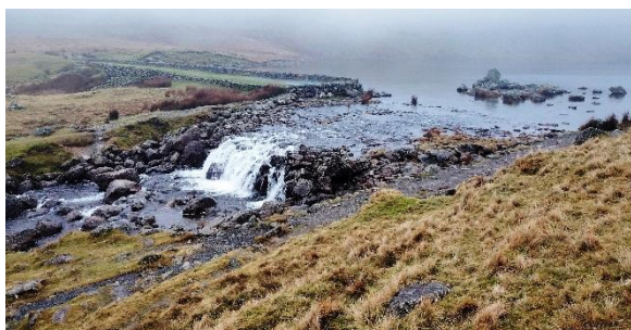
Stickle Tarn spillway and rockfill dam
